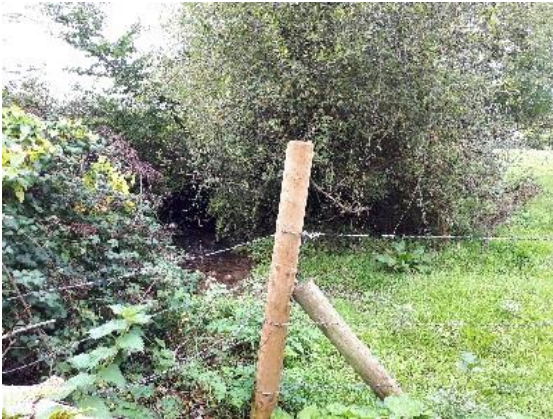
Figure 2: Kilcomma stream downstream of road culvert
