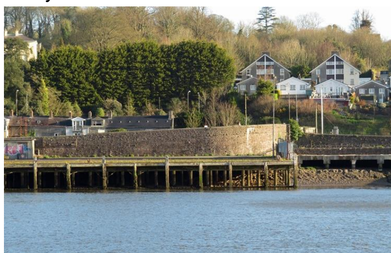
Plate 15.11: Site for bridge landing at Ferrybank
